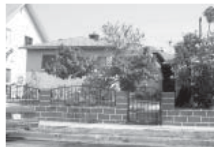
Inappropriate Material Scale
