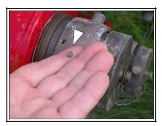
4. Insert a small amount of graphite into the opening between the bearings.
