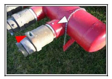
For this FDC model, cover the brass unit set screw with epoxy.
