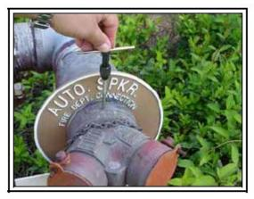
11. Measures the total thickness through the case and pipe thread so that a stainless-steel tamper resistant bolt can be inserted, not to exceed ½ inch into the water flow of the pipe. A tamper resistant bolt is designed to be tightened with a flat head screwdriver but cannot be loosened.
