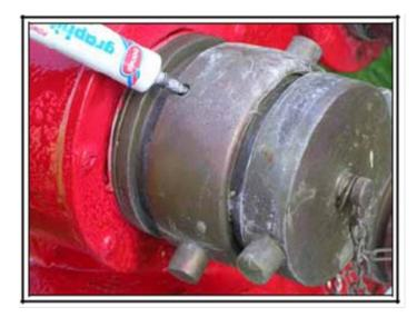
5. Replace the set screw, flush with casing, and spin the connector several times, spreading the graphite. Repeat step 4, as the graphite cannot be forced in one application.
