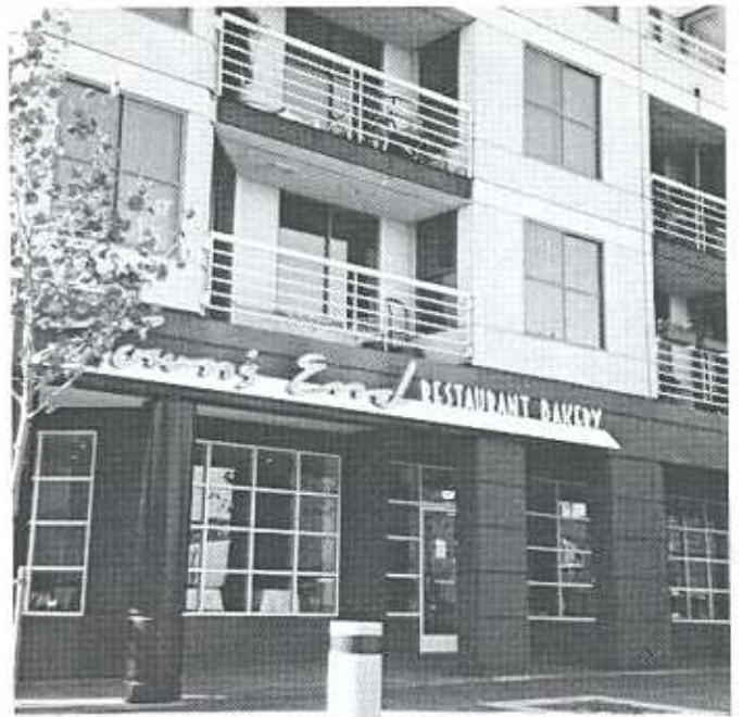
Ground Level Tile or Other Surface for Visual Interest and Ease of Graffiti Removal.
