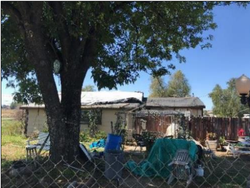
East view of the existing residential structure
