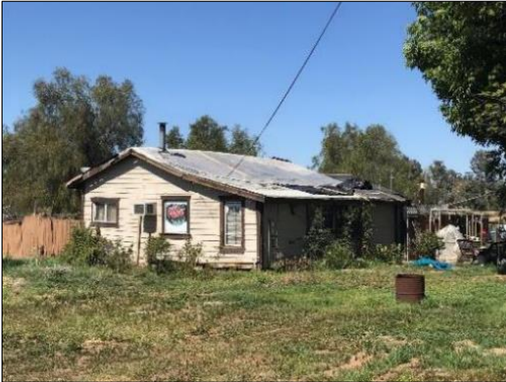
Northwest view of the existing residential structure
