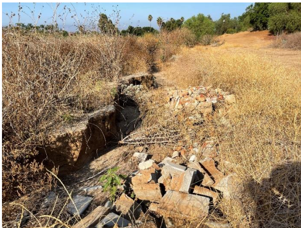
Drainage along southern boundary of site in south-central portion of property, facing west/downstream (09.07.2021).
