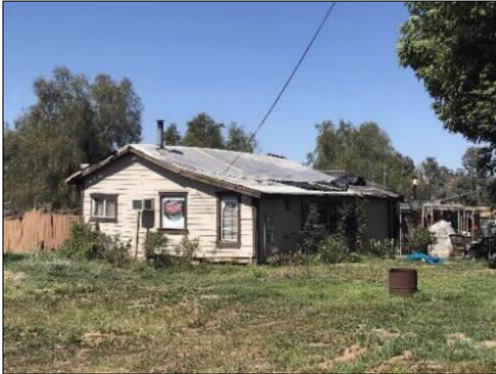
Figure 26. Overview of historic residential home, view northwest
