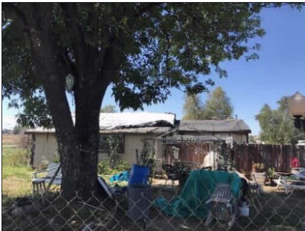
Figure 27. Overview of historic residence, view east
