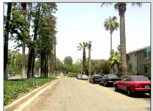
Frontage roads adjacent to Magnolia Avenue have disrupted the historic parkway landscaping in parts of the District.
