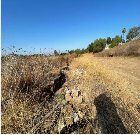
(PP7) Drainage 1 facing west towards adjacent residence
