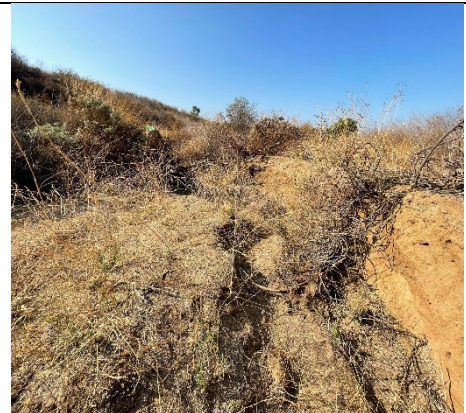
(PP4) Drainage 1 beds and banks
