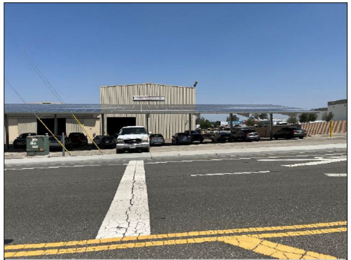
24. Neighboring Property to the North
