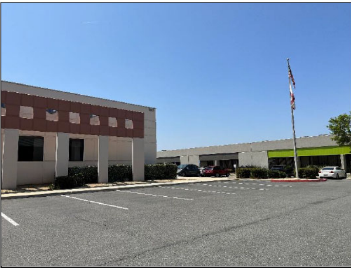
21. Neighboring Property to the South
