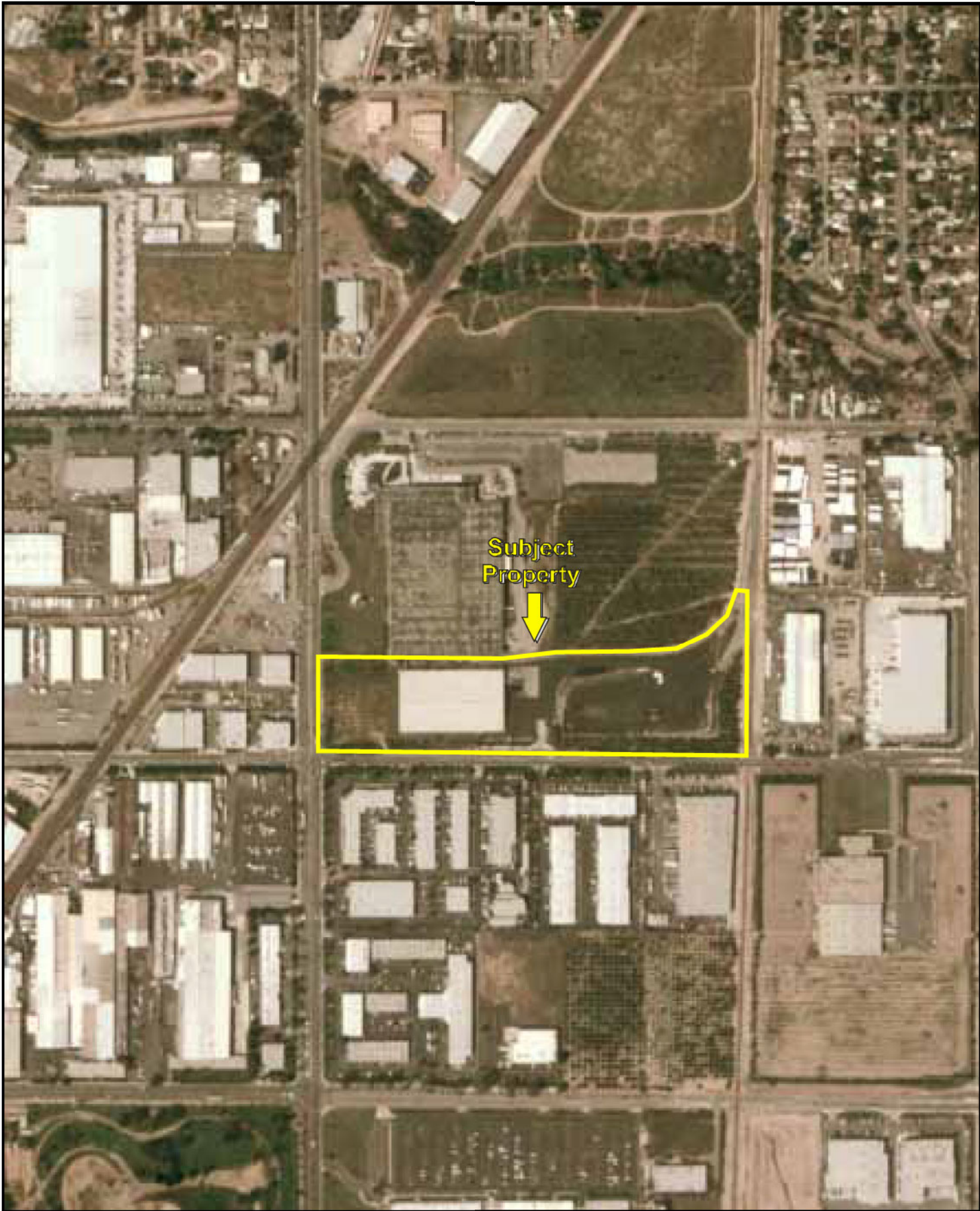
Date of Photograph: 2006
