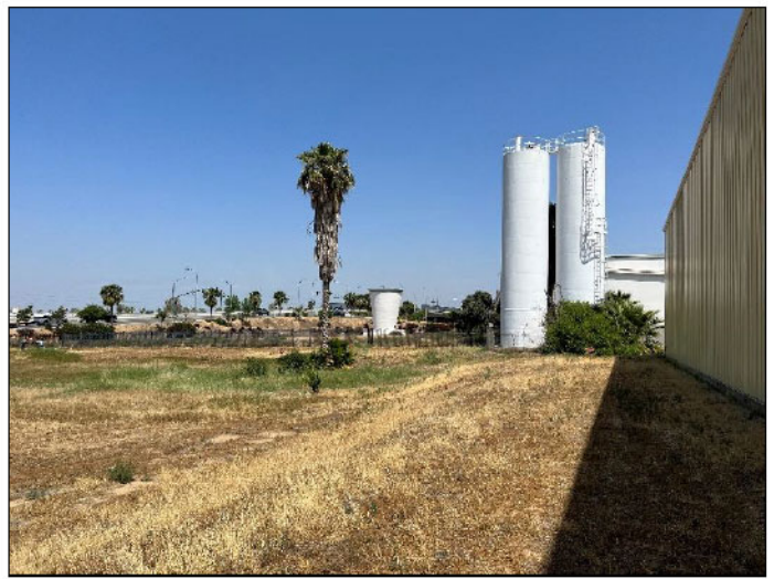
20. Neighboring Property to the North
