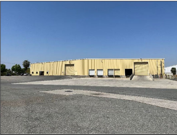
3. Subject Building, looking West
