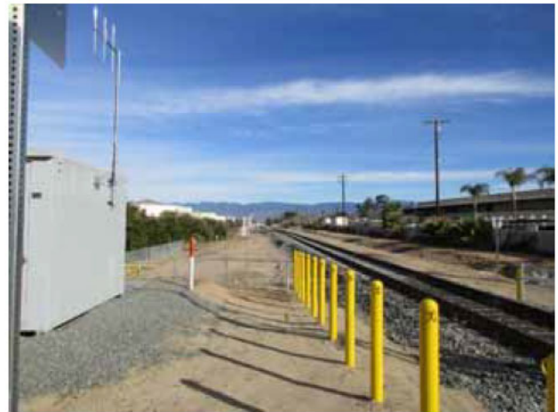
22. View of the railroad tracks and the adjacent property to the east, view facing north.
