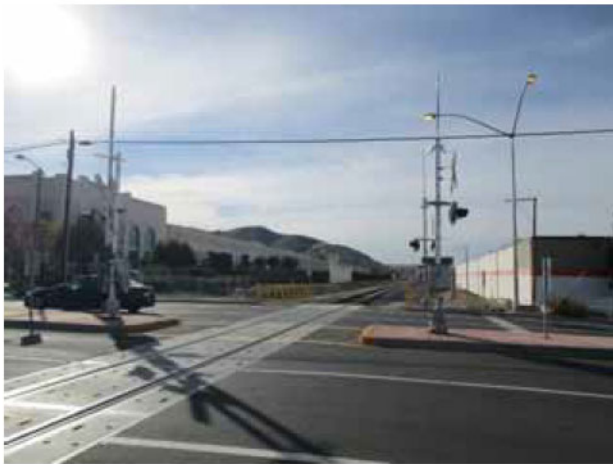
21. View of the railroad tracks and the adjacent property to the south-southeast, view facing south.
