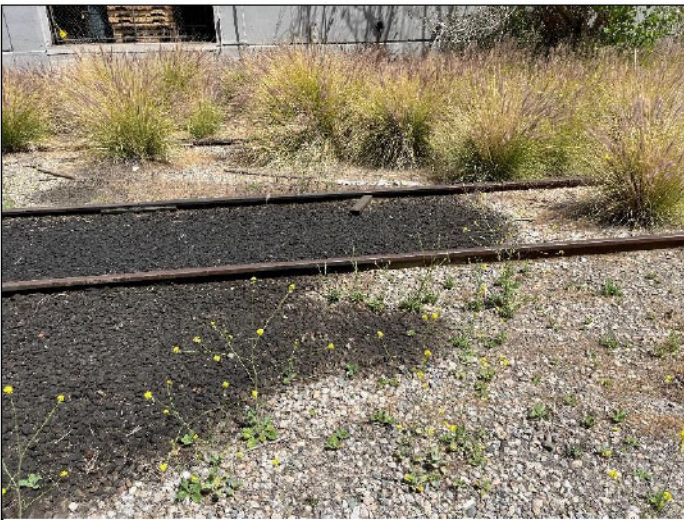
17. Additional Surface Staining at the Western Portion of the Railroad Spur
