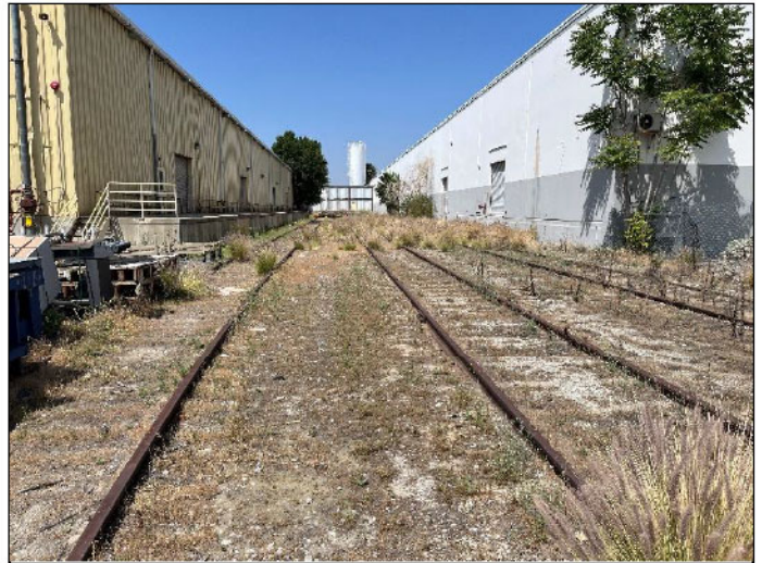
12. Western Portion of the on-site Railroad Spur
