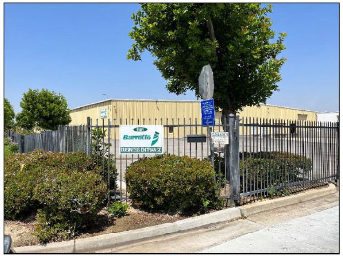
2. Subject Property, 1151 Palmyrita Avenue, Entrance off of Palmyrita Avenue
