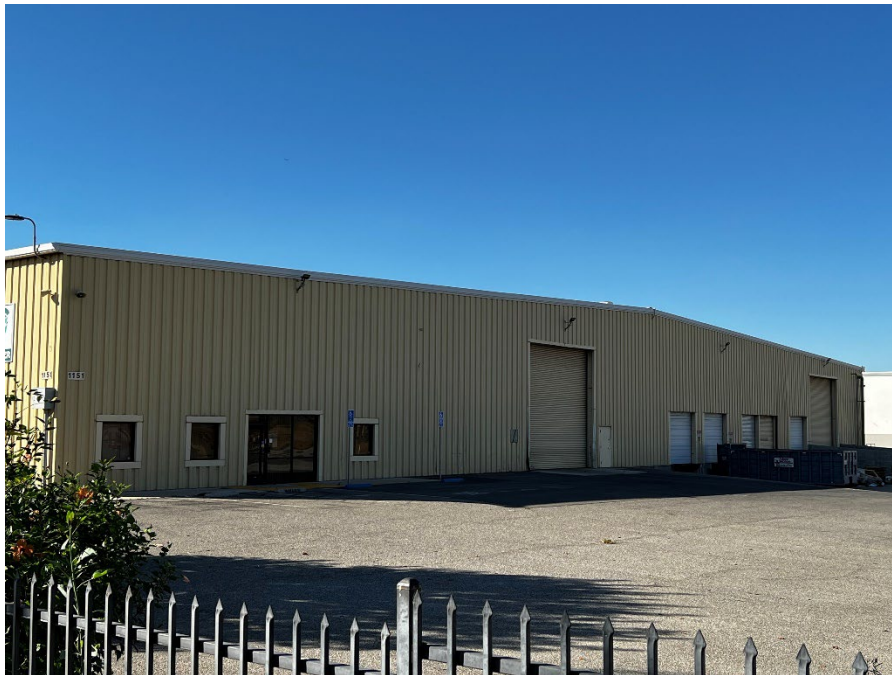
Photo 2: Front face of structure. View southwest.
