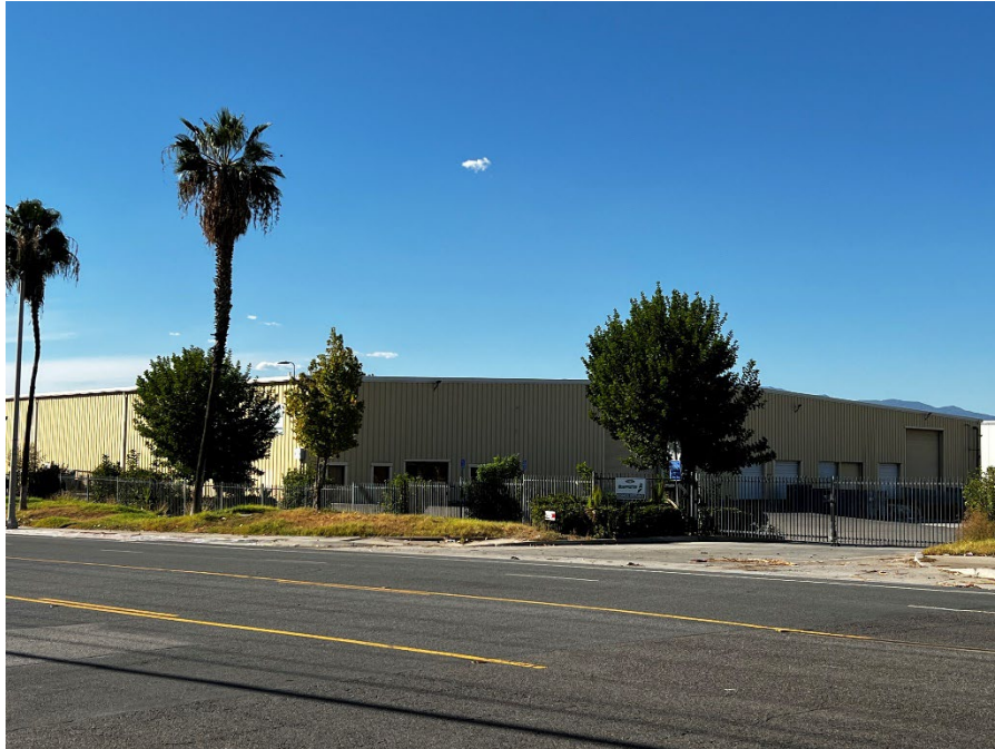
Photo 3: Front face of structure, with view of the left/south face of structure.
