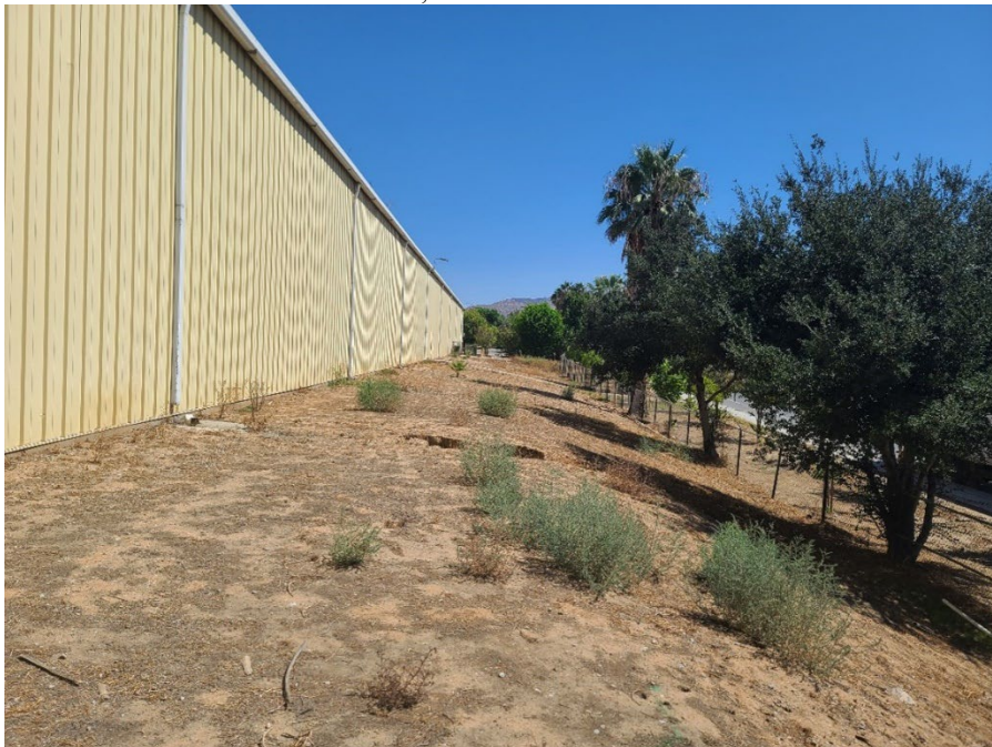
Photo 4: detail of the façade on south face of structure.
