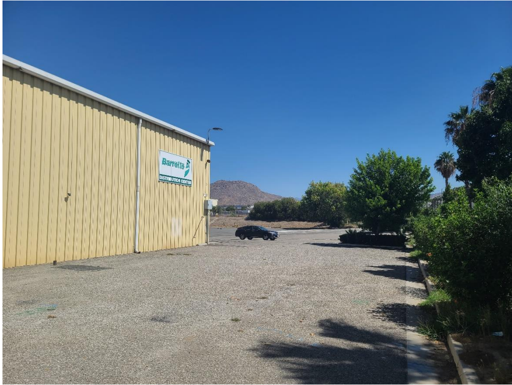
Photograph 1: Overview photo bearing 40 degrees NE
