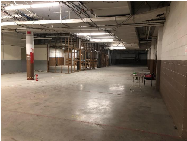
10. View of storage area in the retail structure basement level.
