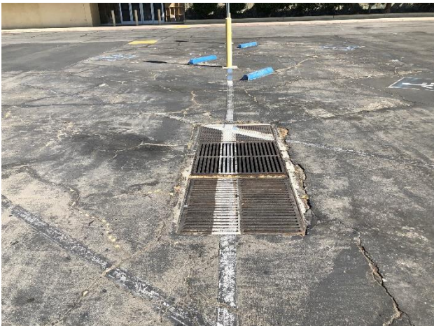
4. View of typical storm drain in the parking area.
