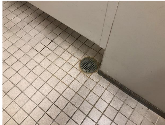
14. View of typical restroom floor drain.
