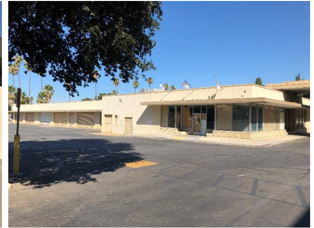
3. View of automotive service center building facing northwest.
