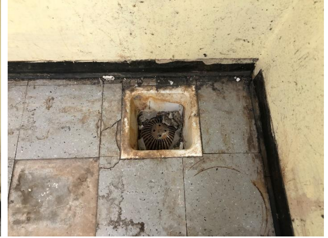
9. View of floor drain in the former maintenance area.
