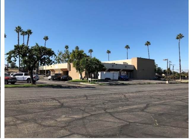
21. View of the adjoining Bank of America building immediately southwest of the Site.
