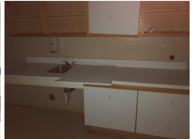
12. View of break room in the retail structure basement level.
