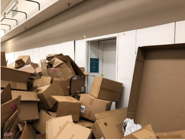
7. View of public elevator.
