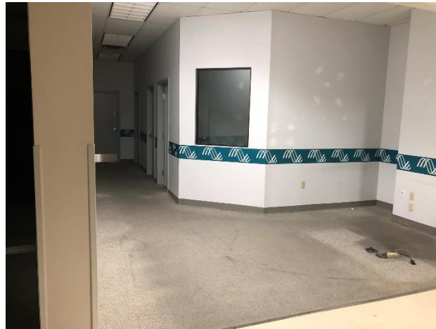
11. View of office space in the retail structure basement level.
